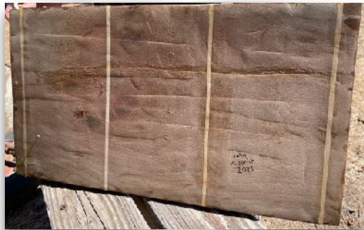
Back of sign showing expansion splines
