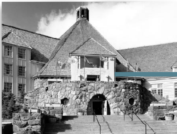
Timberline Lodge entrance, Thunderbird and corbels above the stone entry doorway; Multnomah County Library archival photo
