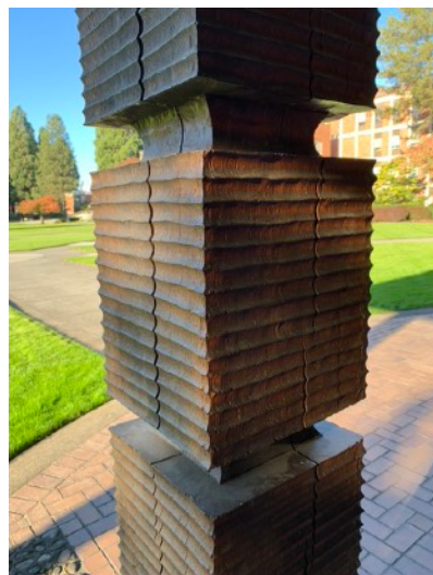
U of Portland Chapel post detail Photo by Larry Wade
